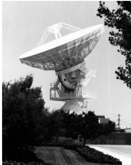
Figure W.2: Satellite-tracking antenna ( Courtesy Space Systems/Loral )
